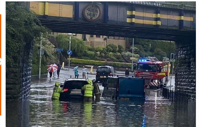
Flooding at Chesser, Edinburgh in July 2020 following heavy rainfall
